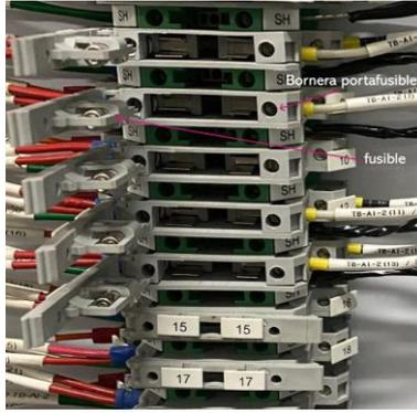
Figura 61. Bornera portafusible.
