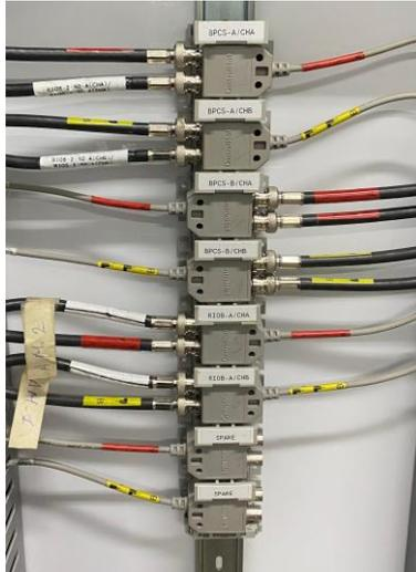
**Figura 58.** Coaxial Straight Y-Tap.
