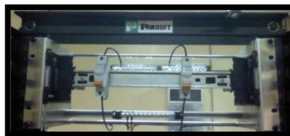
**Figura 126: Switches de -48VDC.**
