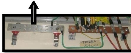
**Figura 74: Barra TGB instalada.**
