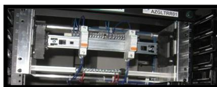
**Figura 197: Switches de -48VDC.**
