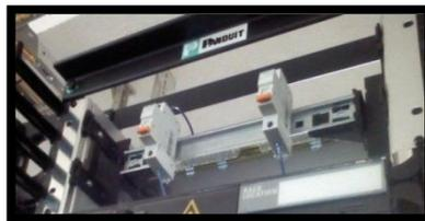
**Figura 227: Switches de -48VDC.**
