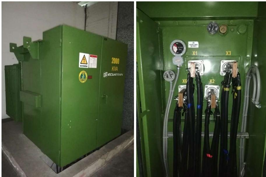
**Figura 68. Transformador Padmounted 2000 KVA**
