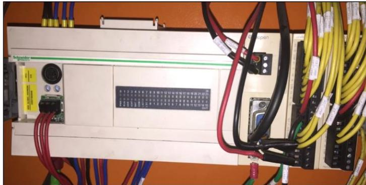
Figura 1.23 PLC Schneider Electric TWDLCAE40DRF.
