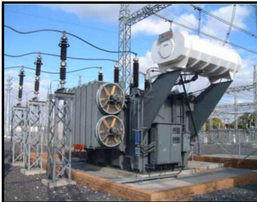
FIGURA 11: TRANSFORMADOR DE POTENCIA [6]
