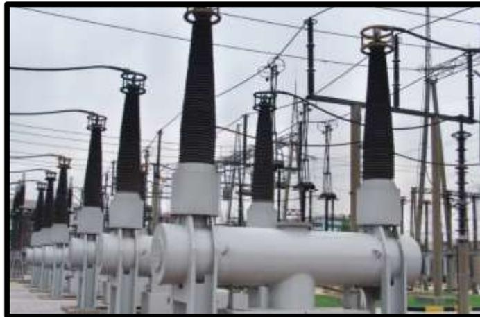
FIGURA 10: INTERRUPTO SF<sub>6</sub> TIPO TANQUE MUERTO [6]
