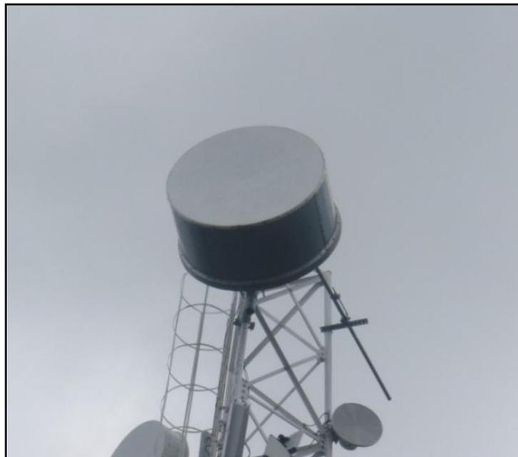
Figura 1.15: Antena Microonda Terrestre
