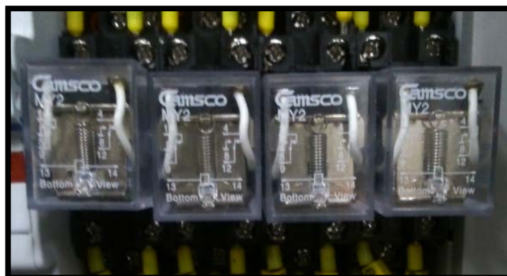
Figura 2.12: Relé de control 10Amp-240V
