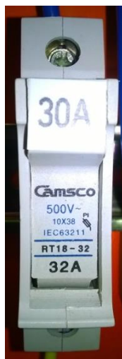
Figura 70: Fusible Base RT18-32
