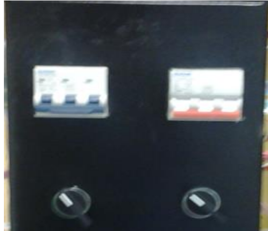
FIGURA 4. 3 Disyuntor principal
