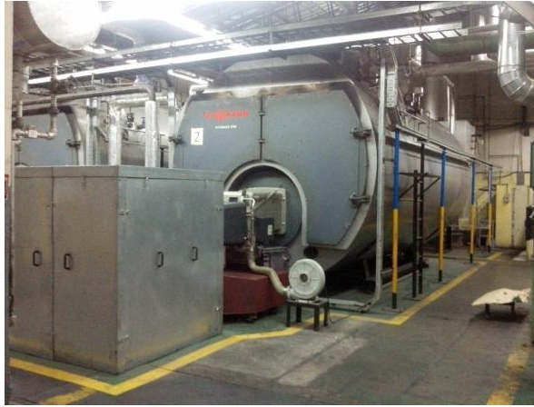
Figura 5: Caldero pirotubular
