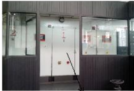
Panel de control
