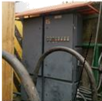
Panel de control
