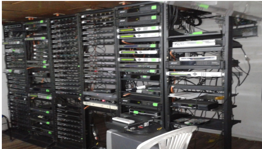
FIGURA 4.1. HEADEND CENTRAL CABLETEL-SERPORMUL 2012
