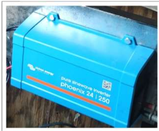
FIG. 16. INVERSOR VICTRON ENERGY 24/250 (AUTOR)
